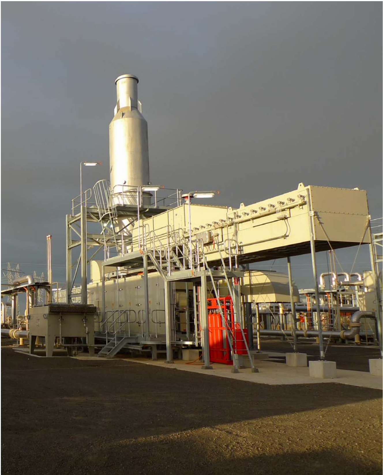
Wollert Compressor Station, Victoria
