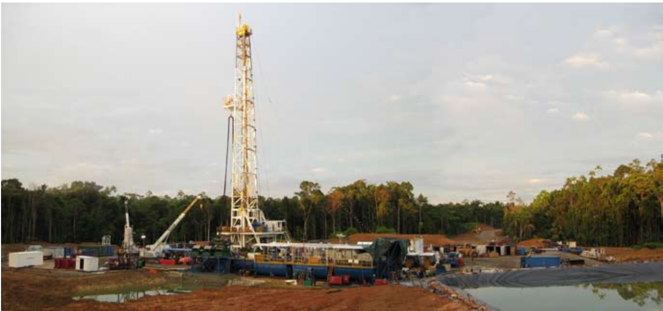
Figure 5.4 Parker Rig 226 at Stanley 2 (Courtesy of Horizon Oil (Papua) Limited)
