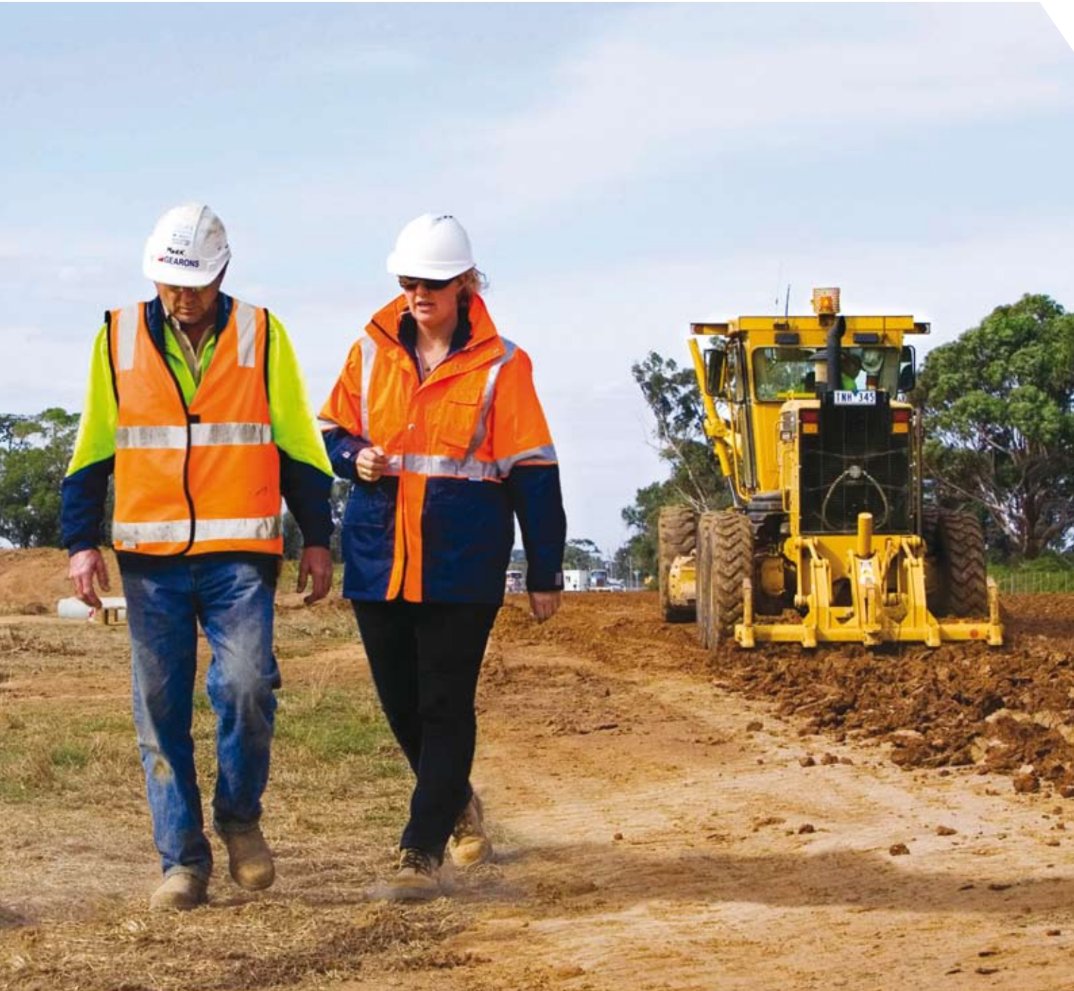
STaPS – Sewage Treatment and Pump Stations, VIC (Baulderstone)
