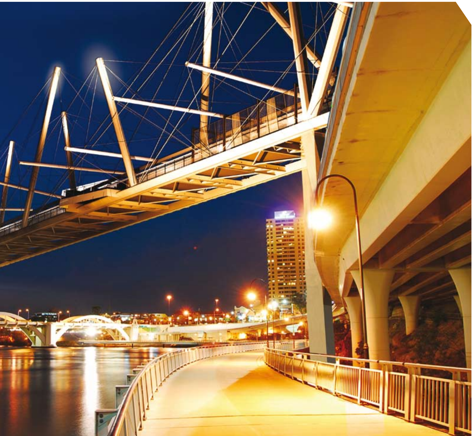
Kurilpa Bridge, QLD (Baulderstone)
