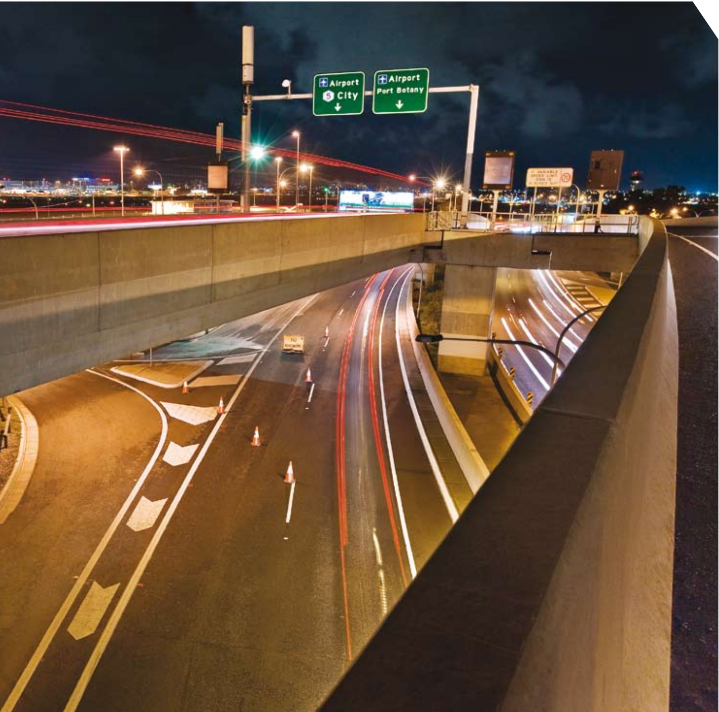
M5 East, NSW (Baulderstone)
