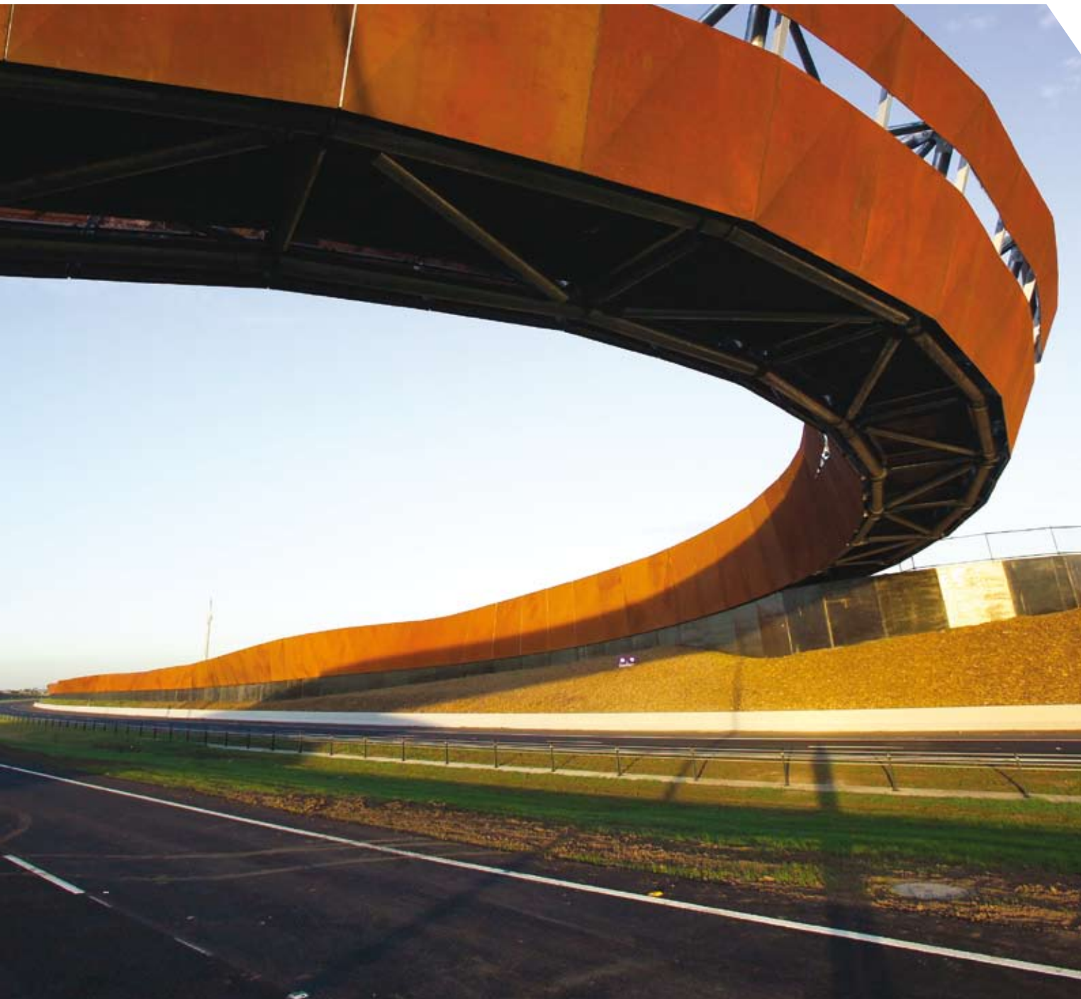
Craigieburn Bypass, VIC (Abigroup)
