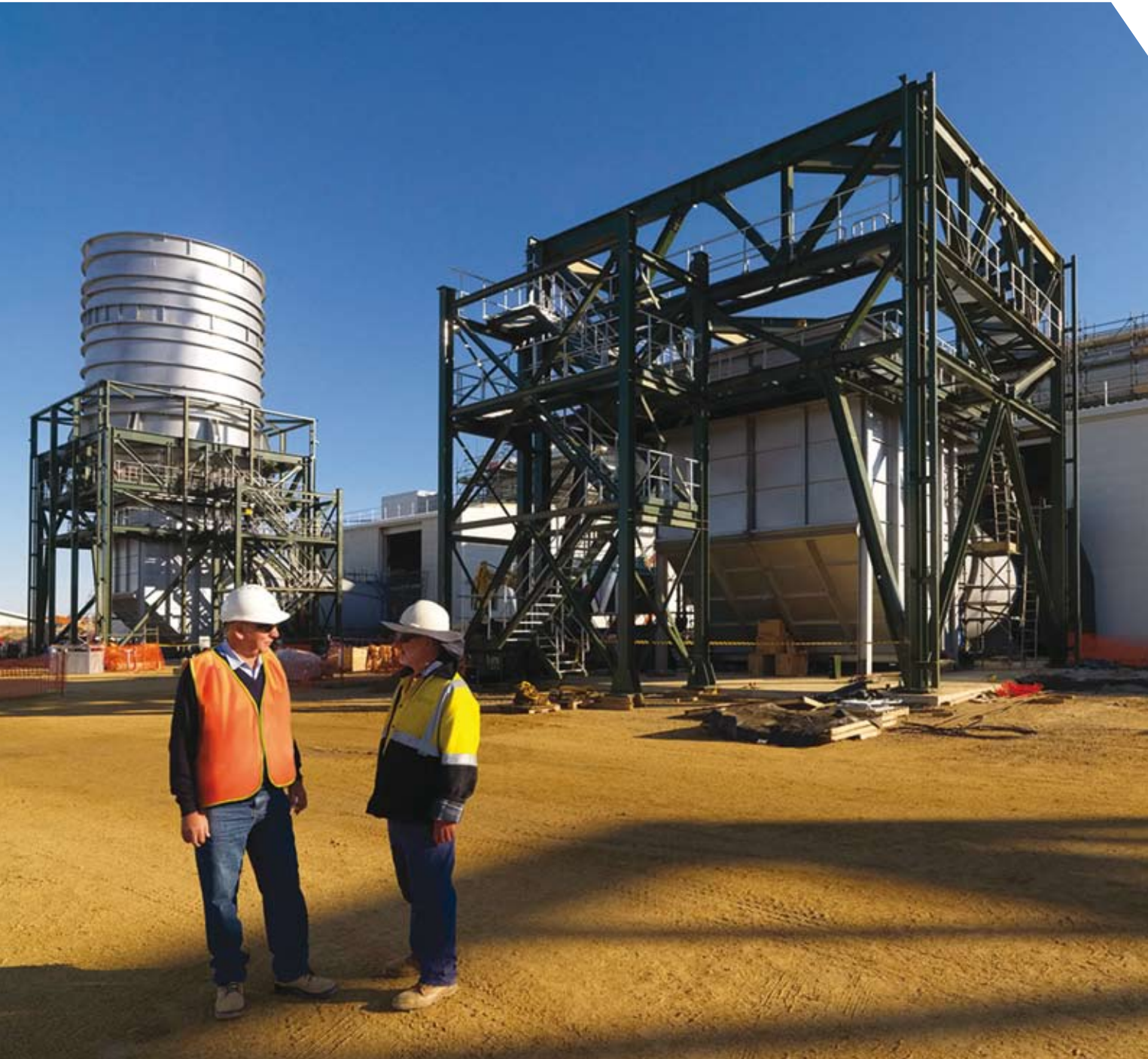
Uranquinty Power Station, NSW (Baulderstone/Conneq)
