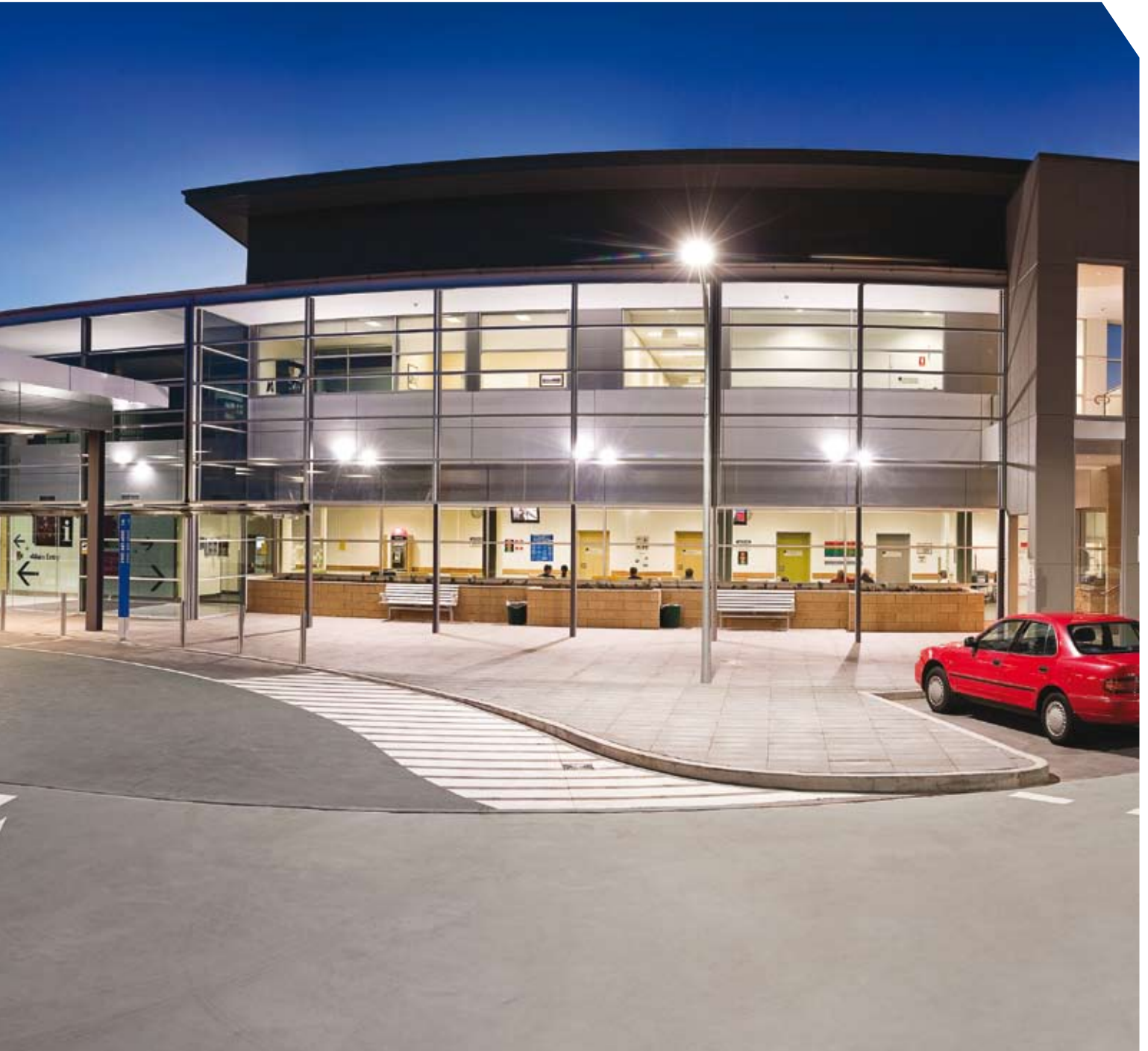
Mater Hospital. Newcastle, NSW (Abigroup)
